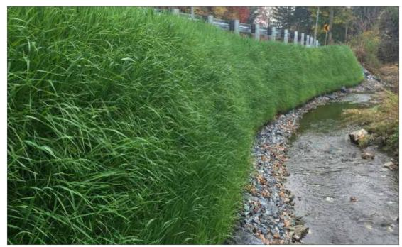
This GreenLoxx® MSE Living Retaining Wall was built for a roadway repair project that increases permeability and green space compared to a concrete block wall. This 2,400 facial square foot wall utilizes 3,300 linear feet of Filtrexx® 12" GroSoxx® filled with Filtrexx Certified™ GrowingMedia™. This wall has the potential to absorb 13,000 gallons of rainfall, per event.
