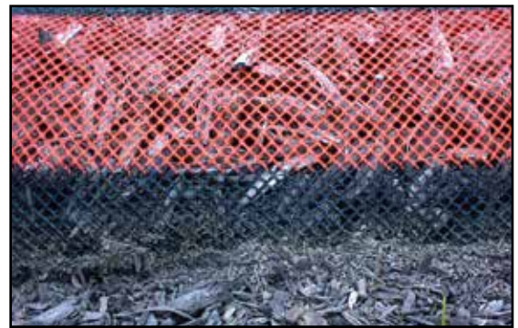
Close Up of Sediment Control
