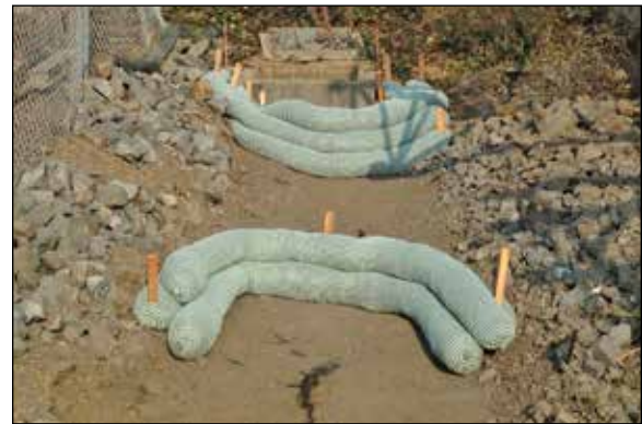
EnviroSoxx used as check dam.
