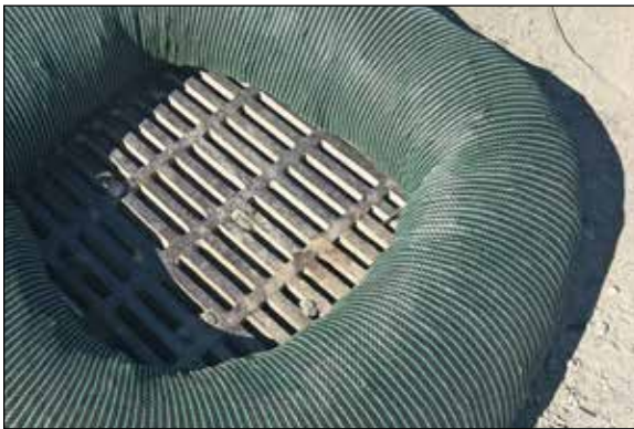
EnviroSoxx used around a drain/inlet.
