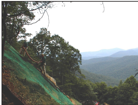
Figure 4.2. LockDown Netting Installation
