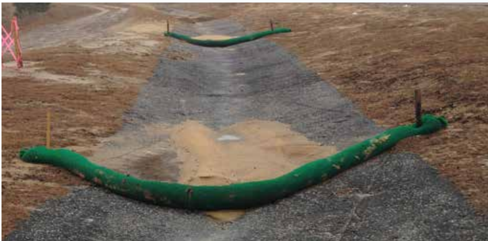
Use for ditch, channel, and swale protection on or near land disturbing activities
