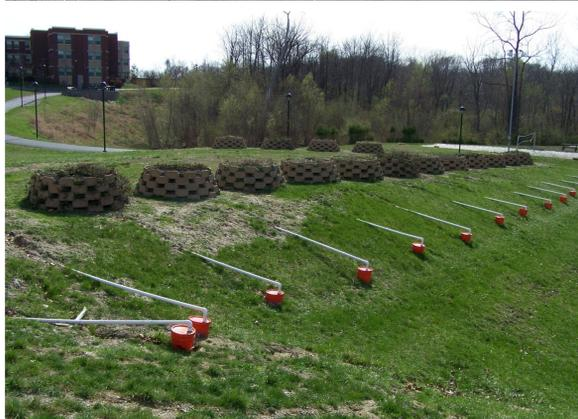
Figure 1. Each wall system is designed with an underlying impervious base layer (top) to direct stormwater through a central water outlet and into stormwater collection units (bottom).
