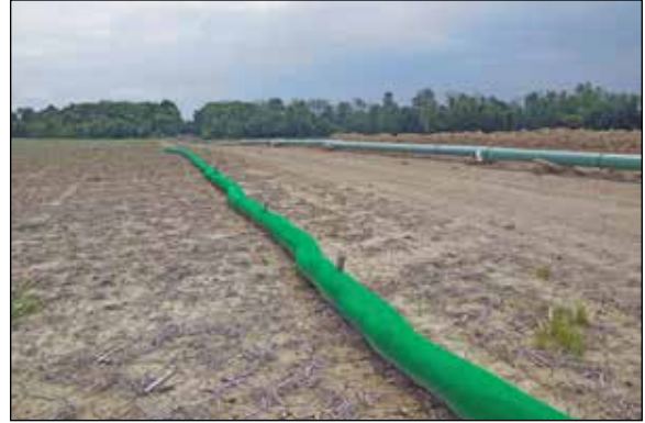
Perimeter Control on Pipeline Project
