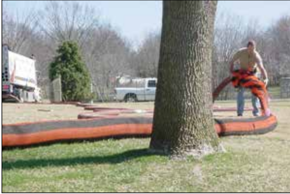
Installation Method – Blower Truck
