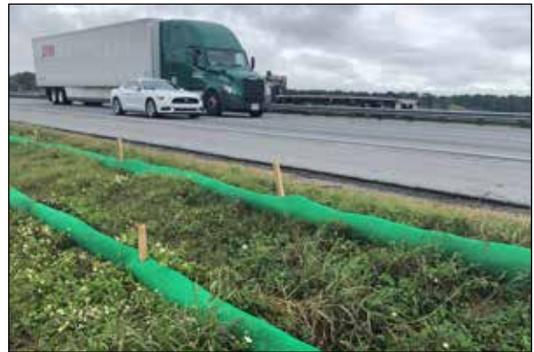
Perimeter Control on Roadway Project
