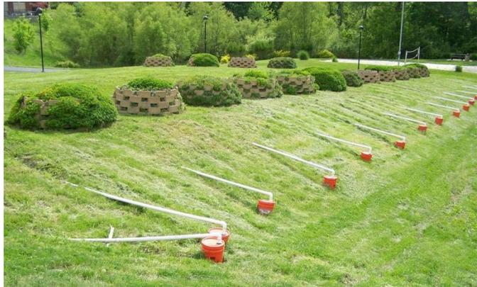
Figure 1b. The green retaining wall systems with 20.4 L collection units (May 2011).
