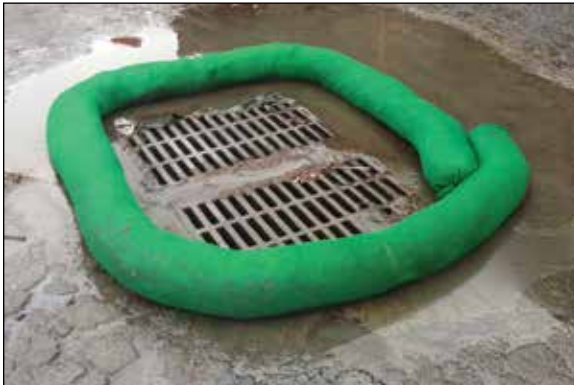
Drain Inlet Protection
