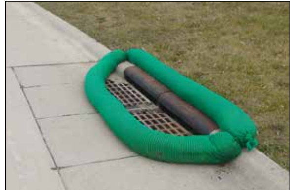
Curb Inlet Protection
