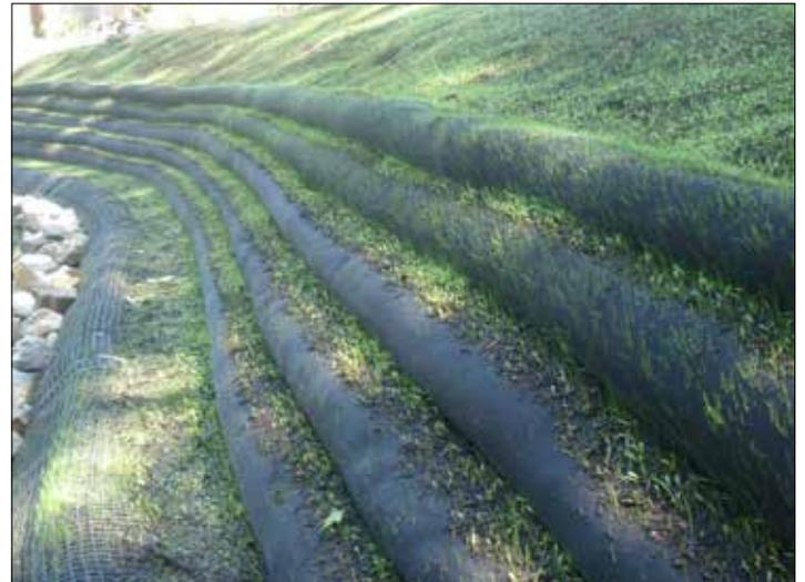
A local Filtrexx Installer engineered a solution to accommodate the stream's highest flow, yet was still attractive during dryer months. The team used 12" Soxx™ to create stepped "flood zones" to minimize erosion, stepping up two feet and back three feet for each level. Above the flood zones they created a LivingWall™ pre-seeded with a deep root grass mix and a wildflower erosion control mix. The solution restored what had been lost to erosion over the previous 20 years.
