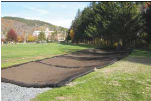
Rain Garden Installed with GroSoxx (Soxx Mesh & GrowingMedia)
