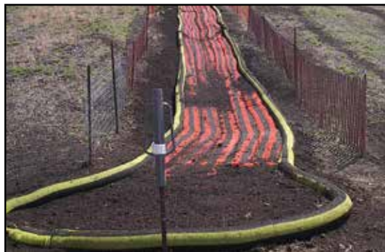
Installation of channel protection
