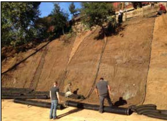
Project site, installation
