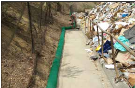
EnviroSoxx at a landfill used as a site perimeter
