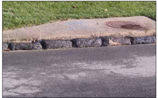
Typical rock bag installation for inlet protection
