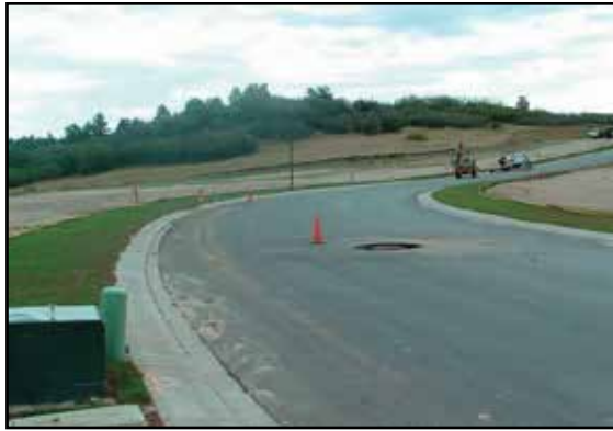
Filter Strip Applied During Construction
