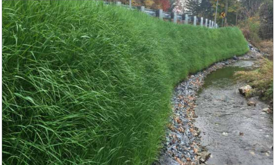
This GreenLoxx® MSE Living Retaining Wall was built for a roadway repair project that increases permeability and green space compared to a concrete block wall. This 2,400 facial square foot wall utilizes 3,300 linear feet of Filtrexx® 12" GroSoxx® filled with Filtrexx Certified<sup>SM</sup> GrowingMedia™.
