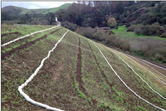
NATURAL ORIGINAL Blower Truck Mesh used as Slope Interruption.
