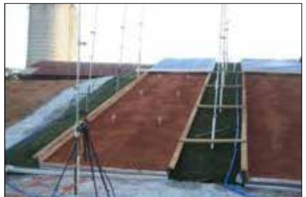
Fig. 1: Test Plot Set-Up Prior to Treatment Installation.
