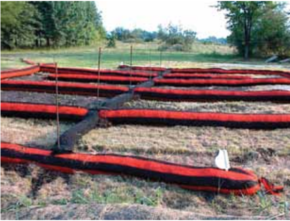
Figure 5 Compost filter sock biofiltration system
