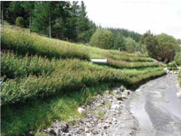
Figure 5 Vegetated compost filter sock
