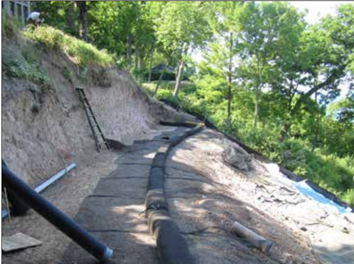
Installation of the GreenLoxx LivingWall
