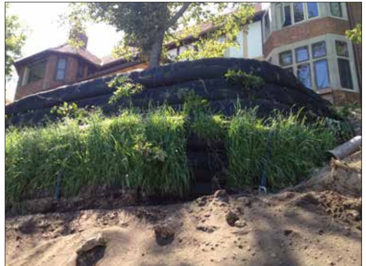
Construction of the upper wall is complete.
