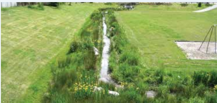
Combines infiltration, biofiltration, and velocity control to reduce stormwater volume and pollutant loading
