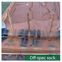
Devices with low flow-through rate, such as off-spec filter sock, overtop faster due to increased ponding & hydraulic pressure behind the device.
