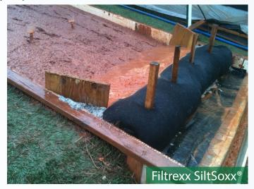
The performance difference between compost filter socks that adhere to federal and state specifications for mesh and media versus those that do not meet these specifications is guite substantial.
