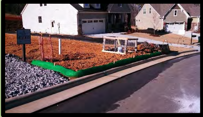
SiltSoxx™ Sediment Control
