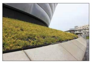
Green Roof Installed with GroSoxx (GrowingMedia + Mesh)
